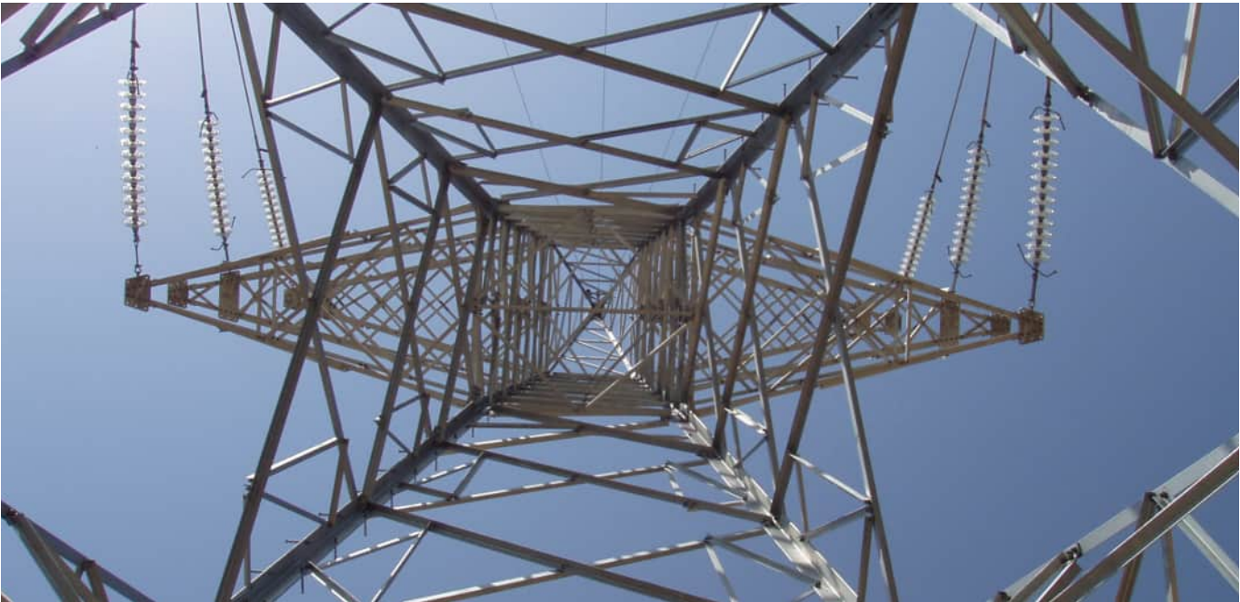
Main protection for lines up to 110 kV
